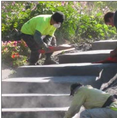
steps in place and prevent heaving, they ran re-bar throughout the section and down into the holes. The next day, the concrete truck would arrive and the pour would start.
