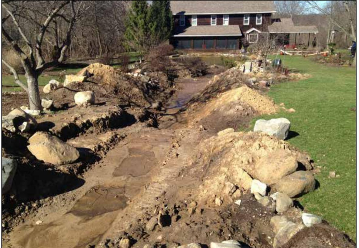
time last season. That has given us a good excuse to rework them and make them better. A pondless waterfall (sometimes also referred to as a disappearing waterfall) is built similar to a pond, but the water goes into a pit filled with rock rather than into a pond. The water is recirculated to the top of the waterfall by a pump located in a vault, hidden in the pit.
